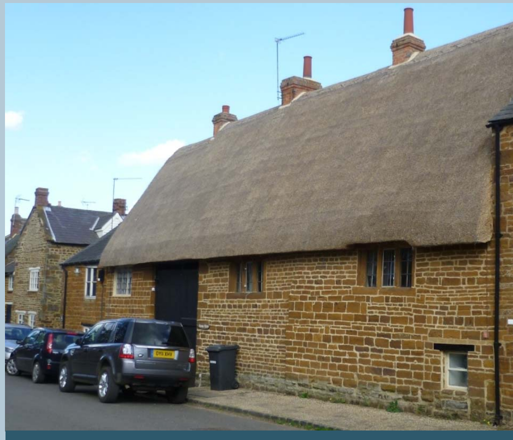
Figure 1: Ironstone and thatch are the vernacular building materials within Eydon .
