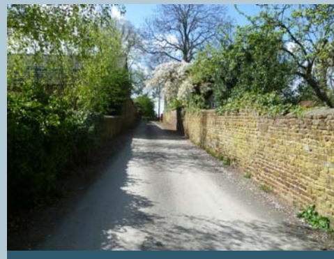
Figure 24: Boundary walls are important
