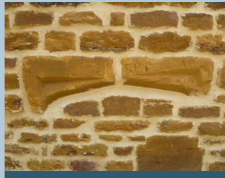
Figure 27: Evidence of historic detailing
