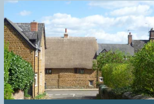
Figure 16: Roofs are mainly slated in Welsh slate, or plain tile. A single thatched roof serves as a reminder of the traditional predominant roofing material in the area.
