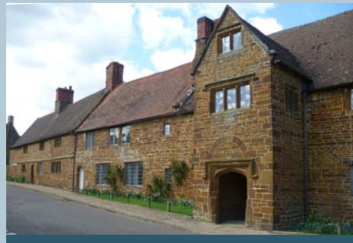
Figure 17: 17th Century stone mullion windows and a four-centred arched doorway with hood moulds over give this building an imposing presence on School Lane.
